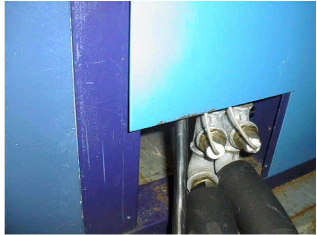
Figure 12- Positioning of the sensors where the cooling water enters and exits the rack.
